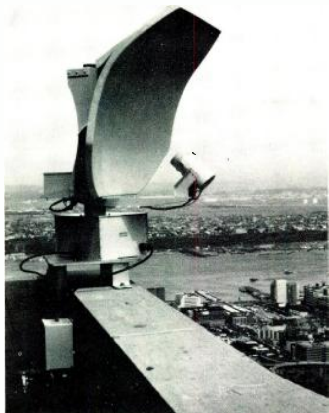
Above, former quad horn system, and below, new Superquad antenna on New York City's Empire State Building, center of WNBC-TV's microwave network.
